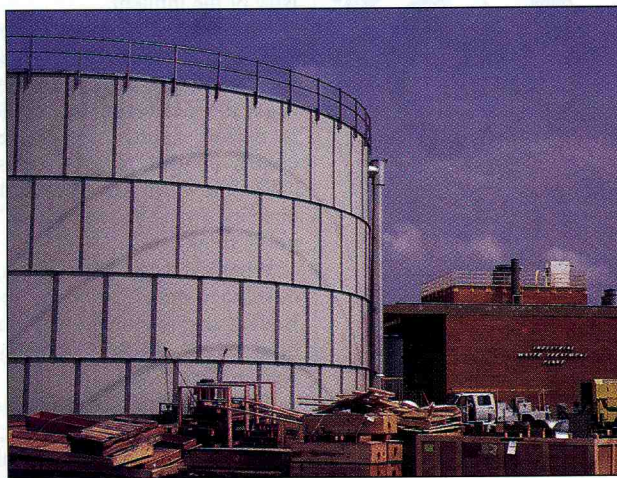
A one-million-gallon, custom-made tank holds water awaiting recycling at Boeing's Wichita plant.
